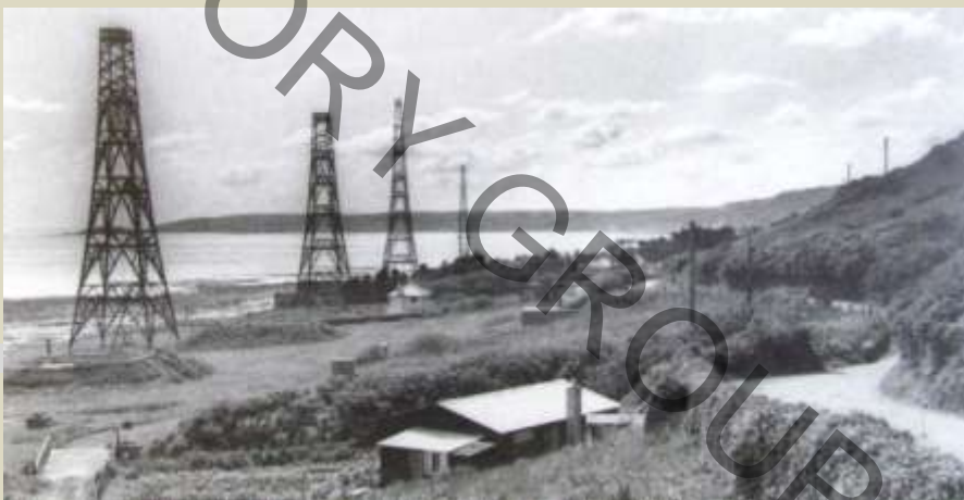
Downderry c 1950s partially demolished radar station
