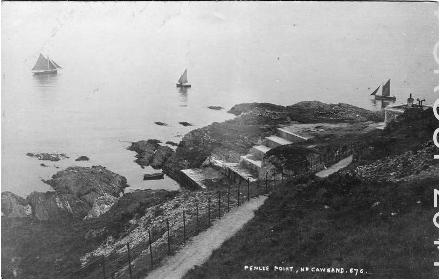
Giant steps at Penlee to land the original 67 ton 13.5" gun in 1892
