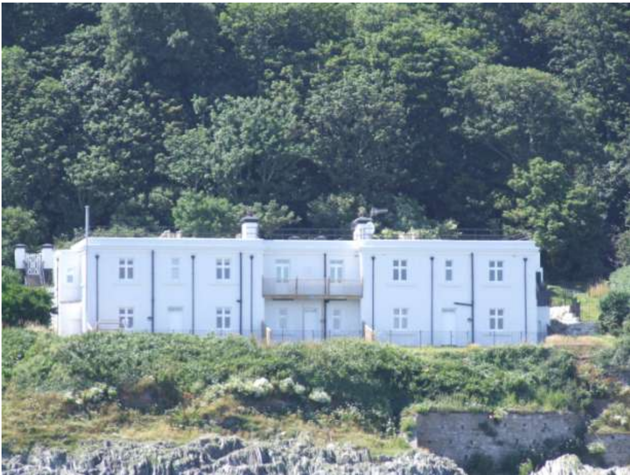
Penlee Fog Station - converted to private accommodation
