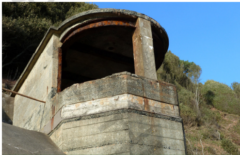
Searchlight (DEL) Housing at Picklecombe
