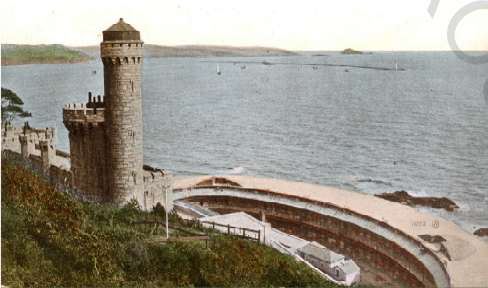
Picklecombe Battery with 'The Officers Mess' in the foreground
